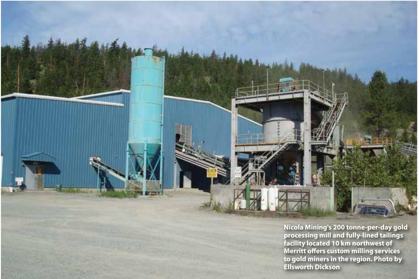
Nicola Mining's 200 tonne-per-day gold processing mill and fully-lined tailings facility located 10 km northwest of Merritt offers custom milling services to gold miners in the region. Photo by Ellsworth Dickson
